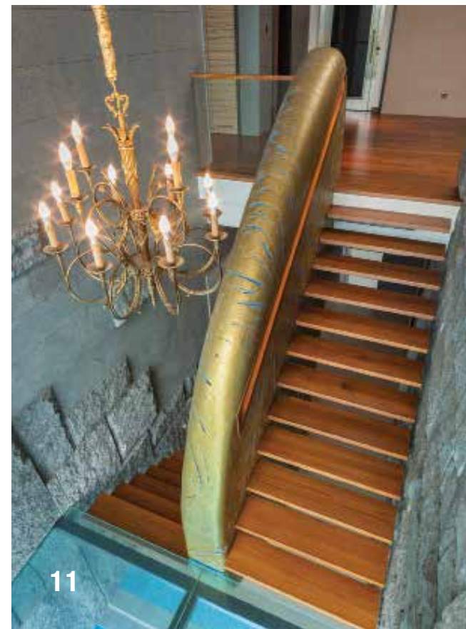
[8-11] The central staircase features a hand-painted concrete wall, cantilever steps and a glass landing that hovers over the swimming pool below. [12-13] The verandah overlooks the swimming pool.
