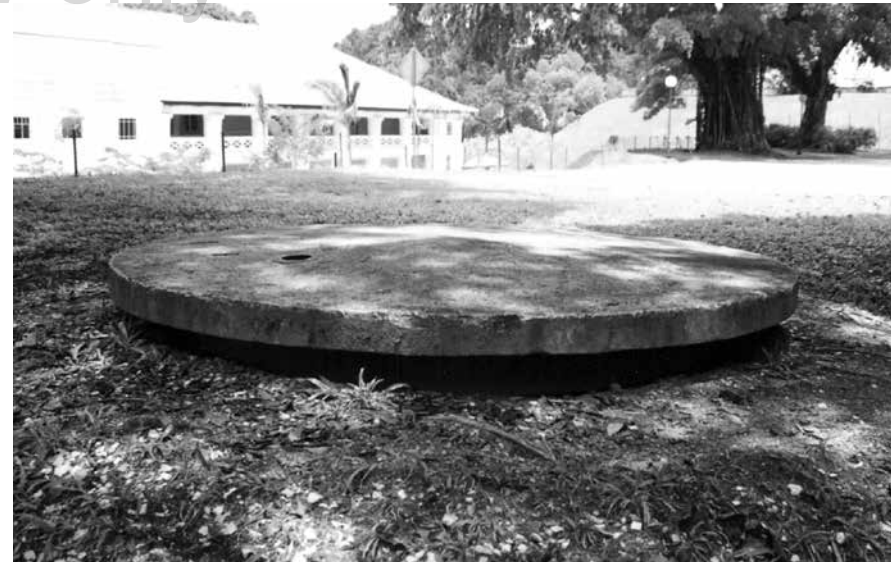
The only identifiable signs of the Battlebox from the top of Fort Canning Hill, the concrete mushroom-like structures formed the top of the ventilation systems operating in the complex below. The mushrooms still remain in the park, in addition to a new structure above the emergency rooftop exit. In the background is the former barracks on Cox Terrace. It has now been converted into an arts centre and a culinary institute.
