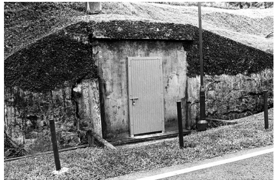
The locked door on the Dobbie Rise side of the bunker, before the lock accidentally fell apart. It could easily be mistaken for a storage shed. Note how close it is to the main road on Dobbie Rise and the drainage ditch dug in front of the doorway.
